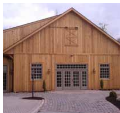
Two 12' AirVolution fans are at the center of a ductless climate system at Glasbern Inn's newly-renovated barn.
